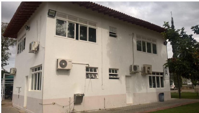
Bloco A – fachada frontal
